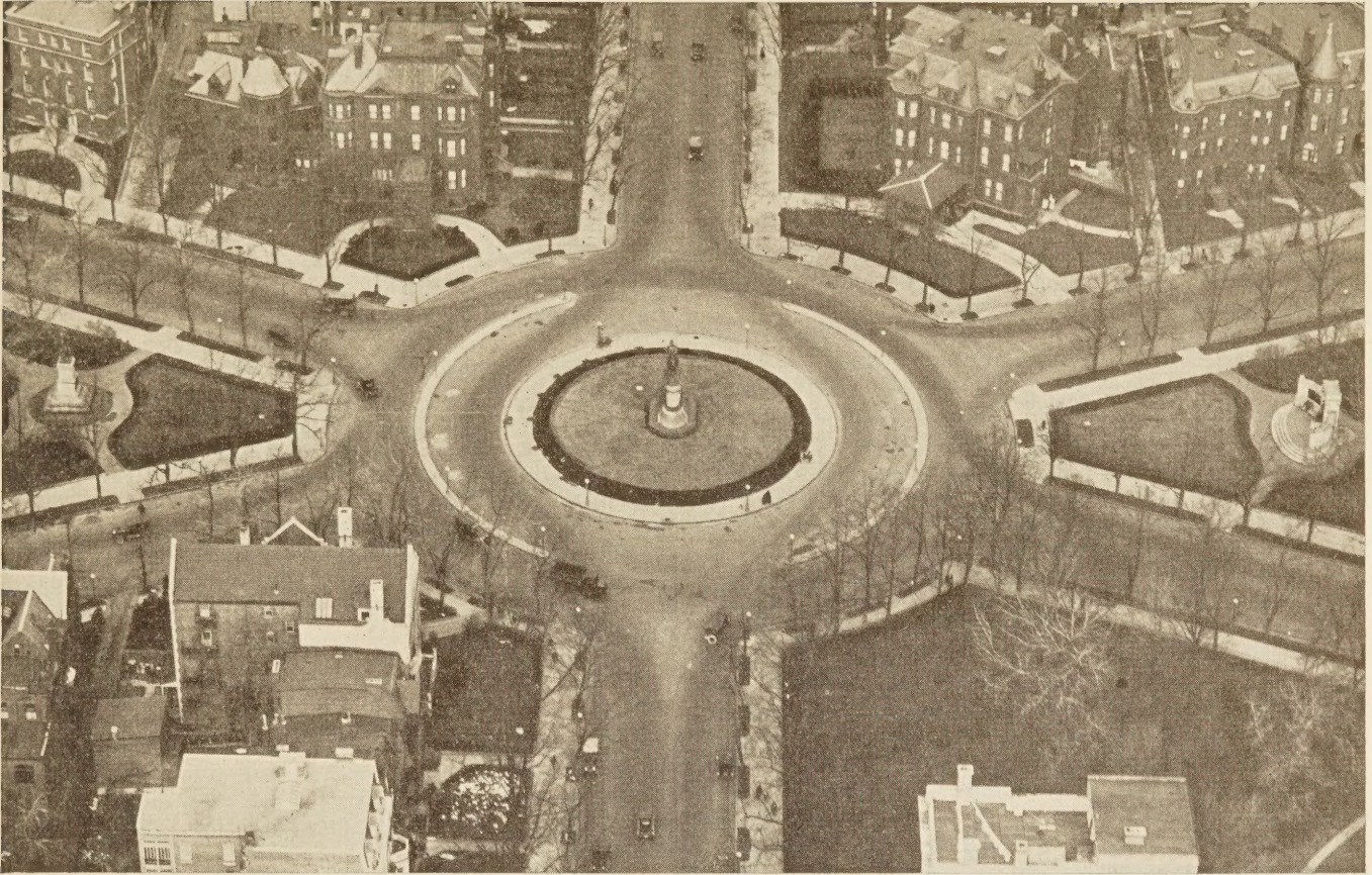
FIGURE 5.—VIEW OF SCOTT CIRCLE, WASHINGTON, D. C., SHOWING AREAS UNUSED BY TRAFFIC AT ENTRANCES OF CONVERGING STREETS
